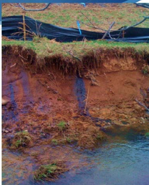
Drill site, Harrison County, WV. Landowner reported seeing oily substance bubbling up from ground and into stream. Driller later cited for putting a well pad on top of a wetland area.
