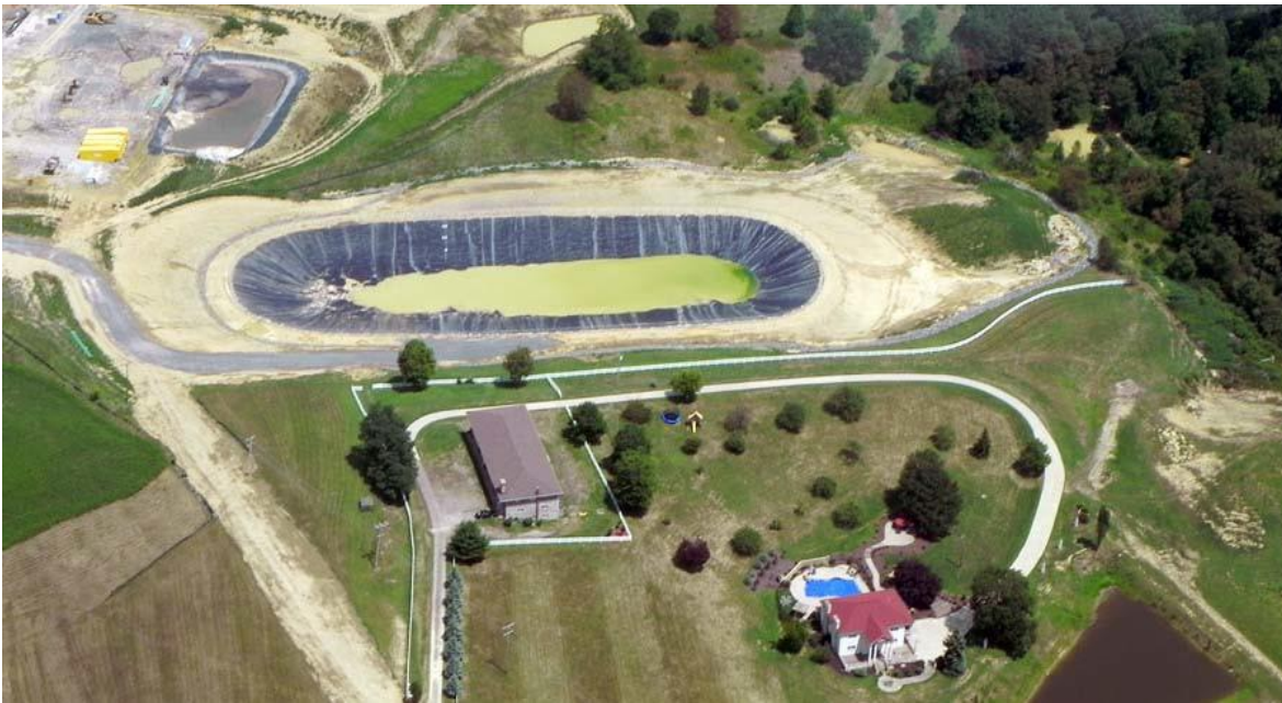
A hydro-fracking drilling pad and storage pond in Pennsylvania show the proximity to the homeowner's house as well as the large scale of the operation. (Source: Steve White/MarcellusProtest)
