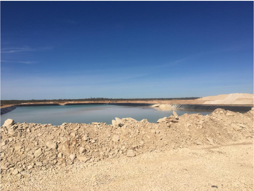
Photograph 5. Sludge Thickening Basin
